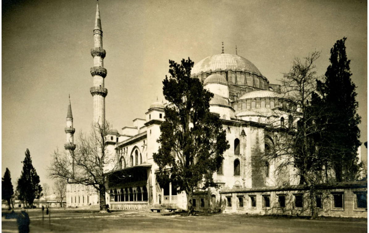
PLATE 20. Süleymaniye Mosque in Constantinople (Cat. No. 61b). This mosque was commissioned by the well-known Sultan Suleiman the Magnificent and built by his architect/engineer Sinan Agha between 1550 and 1557. Mimar Sinan was one of the greatest and celebrated of Ottoman architects and is responsible for the planning of a large number of mosques, schools and palaces.
