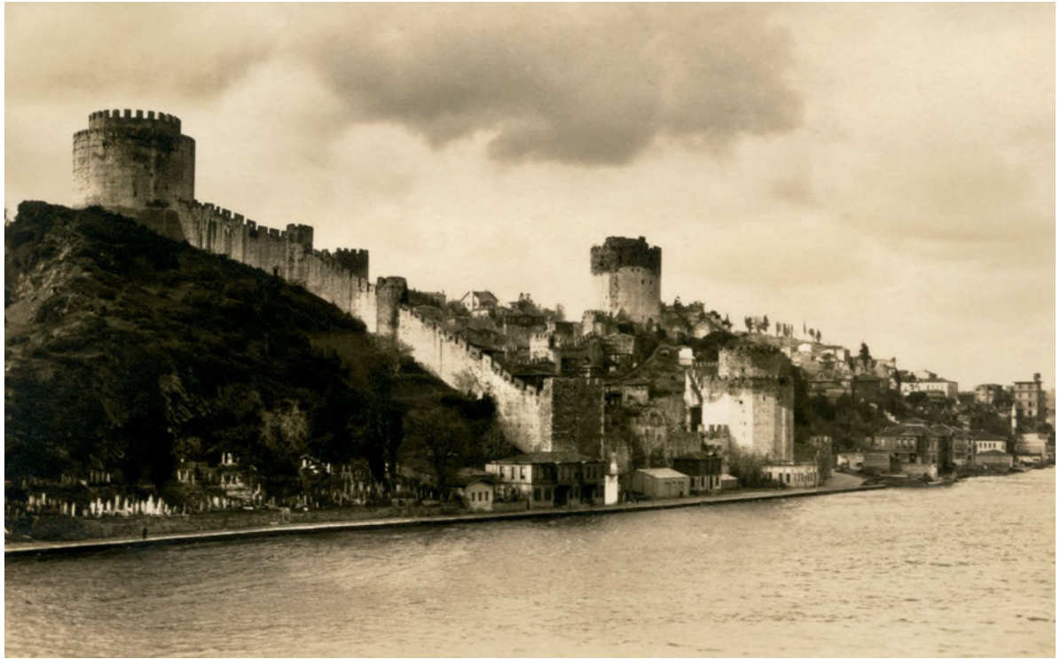
PLATE 25. The fort of Rumeli as seen from the Bosphorus (Cat. No. 63b). Strategically situated on one side of the narrow straits, this fort consisting of towers and curtain walls, was built in 1452 to defend the entrance to the Bosphorus. Any ship approaching the straits could easily be fired upon from the fort. This view of Rumelihisari has not changed very much, though the fortifications today are in a much better state of repair.
