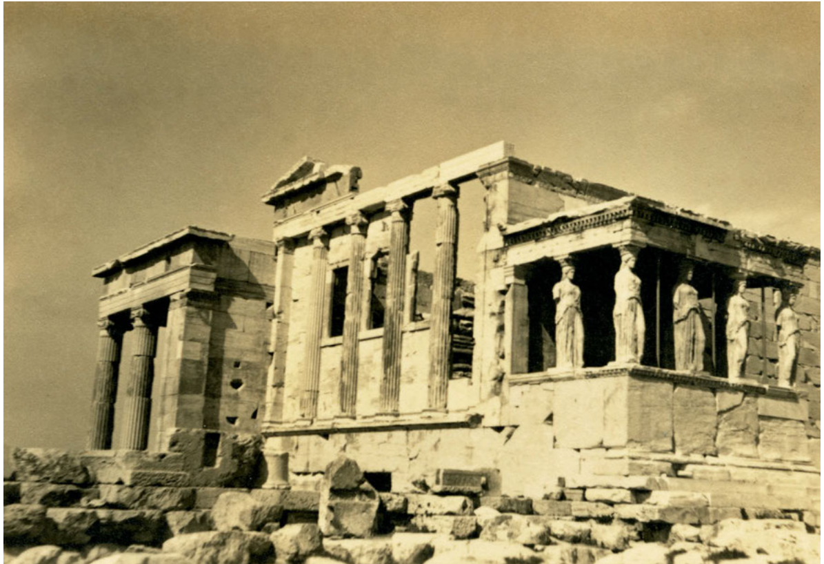
PLATE 10. The Erechtheion and the Porch of the Caryatids (Cat. No. 27b). The Erechtheion is a temple dedicated to the gods Athena and Poseidon and it is situated on the Acropolis. On the right is a porch with its ceiling supported by six sculpted draped female figures (Caryatids) instead of columns. One of the original six figures was removed by Lord Elgin in the nineteenth century and is in the British Museum, London.
