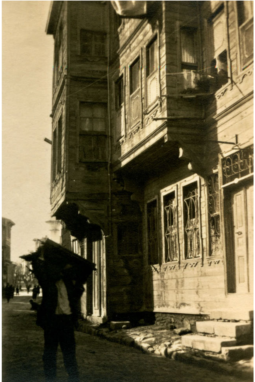
PLATE 23. A timber house at Constantinople (Cat. No. 18b). The traditional timber house of Constantinople is an important feature of Turkey's rich cultural heritage. They were originally built because the city is situated on a seismic fault, and they are less susceptible to collapse. However, their present-day conservation is incredibly difficult.
